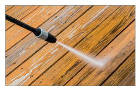
What can happen with high pressure power washers is that some of the water will push itself out through the deck system and cause leaking. This is usually not a permanent problem, and the system will return to normal functionality (leak free) when you're not using the power washer.
