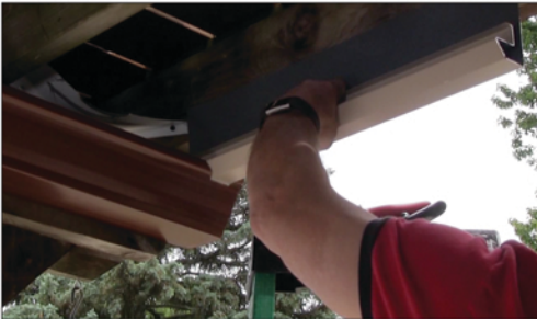
Use Side Cap to cut the notch in the Gutter
