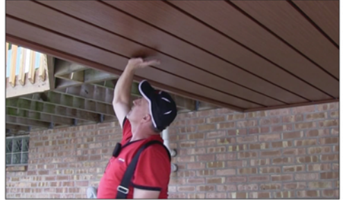
Gently slap the last Panel into place
