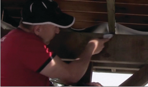
Clean the gap below the joist with a wire brush
