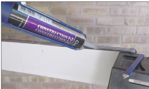
Run a bead of Sealant along the back tab
