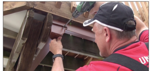
Attach the End Cap to the Side Cap with a Zip Screw
