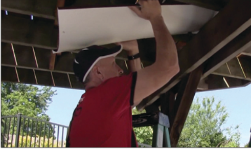
Slide your pan flashing up over the beam
