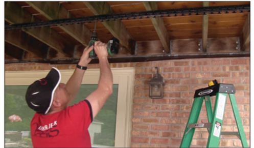
Temporarily secure the Carrier to the joist
