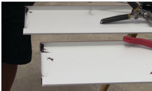
Seal the boxed end with your sealant
