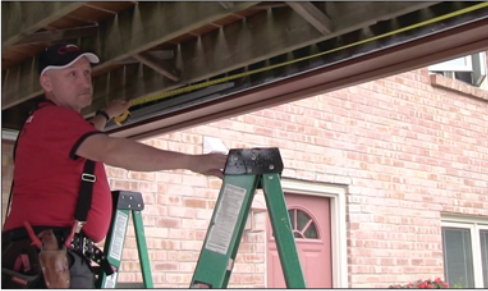
Measure the spacing for the Carriers
