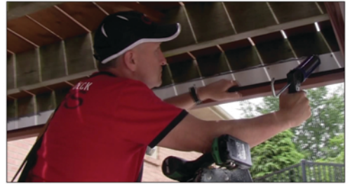
Secure and seal the Side Cap
