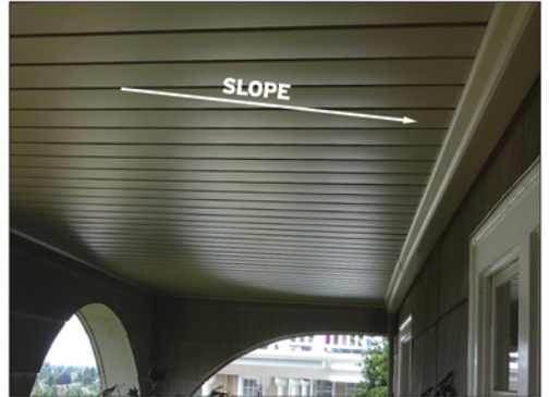
Slope direction is toward the house, away from the beam.
