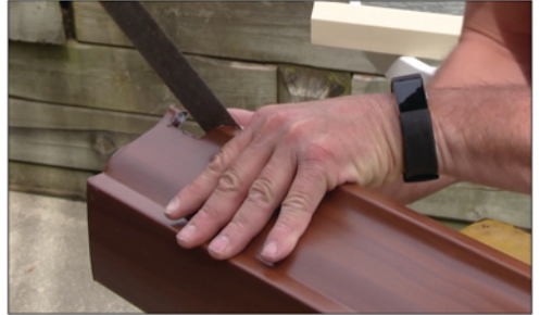
Remove any aluminum burrs with a file
