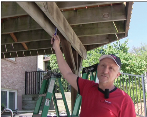
Open beam deck construction.
