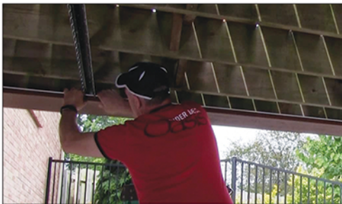
Put the Panel into the Alignment Carrier
