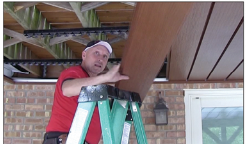
Gently slap the last Panel into place
