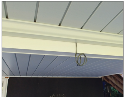
Open beam wrapped with composite decking.
