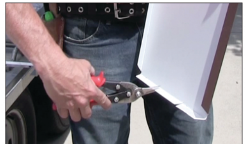
Put two cuts in the bottom tab to allow for proper cupping
