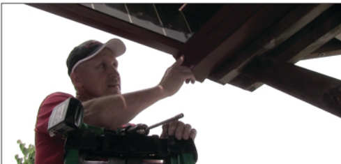
Tighten up the “give” between the Side Cap and the Gutter
