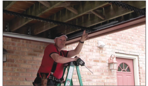
Secure the Carrier at the closest joist
