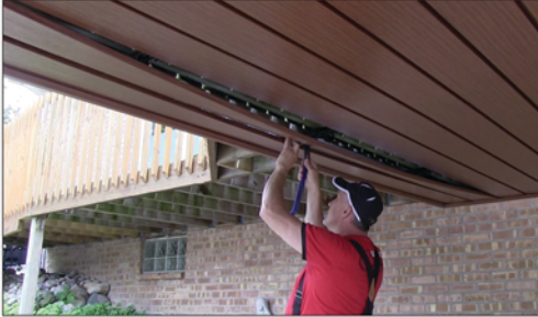
Use a flat bar to secure the final Panel
