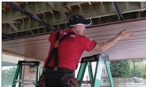
Snap the Panel into the Carrier, then secure it with a gentle slap
