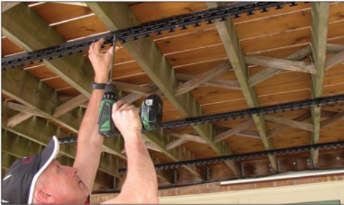
Secure the Carrier 4 or 5 joists away from the first Panel
