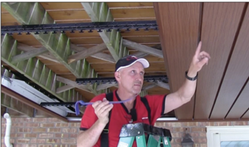
Use a flat bar to secure the final Panel
