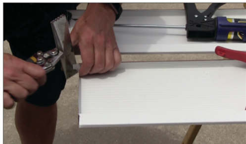
Cut tabs on one end in order to create a “boxed end”
