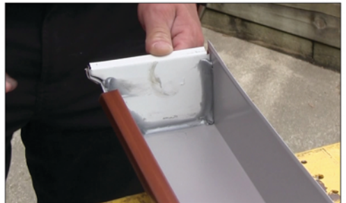
Secure and seal the end cap
