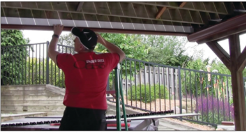
Slide the Side Cap into the notch in the Gutter
