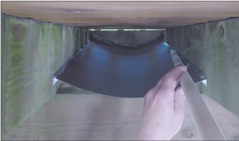
Seal your pan flashing
