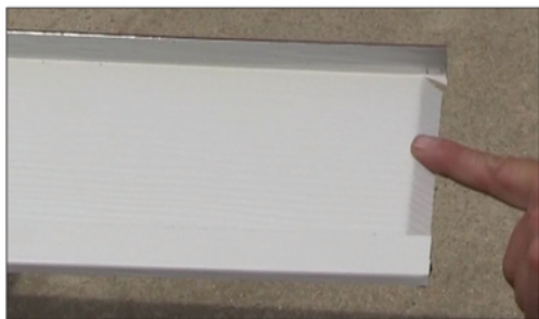
The other end needs a lip to allow water to flow into the Gutter
