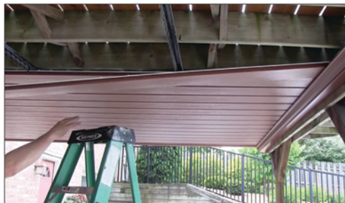
Slide the Panel into the Gutter, then back into the G-channel
