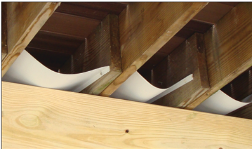
Pan flash between every joist
