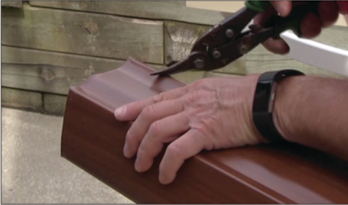
Cut the notch out the Gutter with your snips
