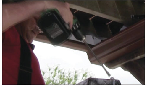
An 8" drill bit makes it easier to get over the gutter
