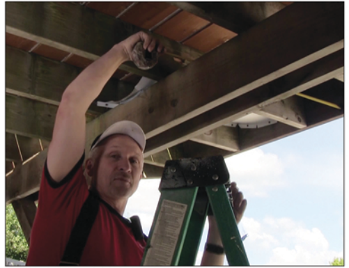
Measuring the pan flashing length
