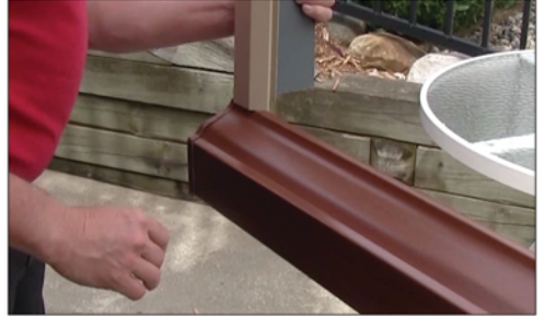
Use the Side Cap to create a stencil on the Gutter
