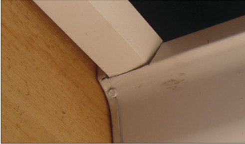
The Side Cap needs to rest in a notch in the Gutter
