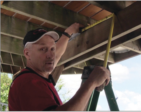
Measuring the pan flashing width
