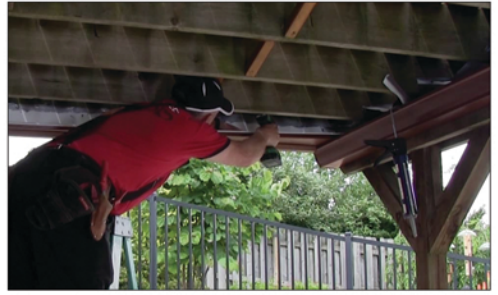
Secure the panel to the Side Cap
