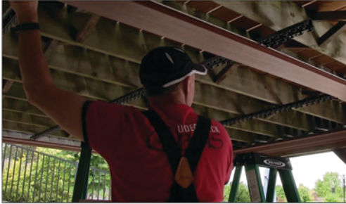
Set your TEST Panel to determine Carrier pitch
