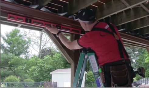
Set the pitch from the high end to the center
