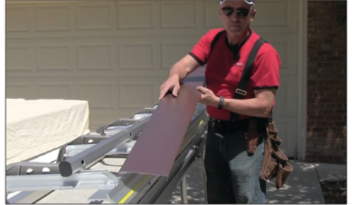
Create a 15° drip line on the other side
