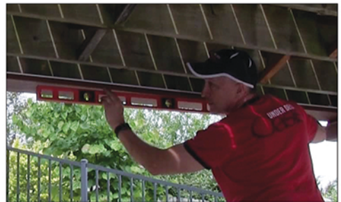
Use your level to ensure proper pitch
