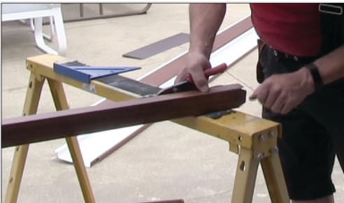
Create fold tabs in the G-Channel
