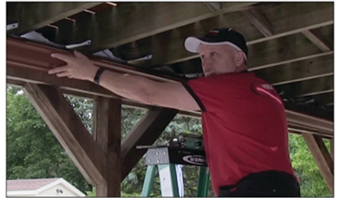
Adjust the pitch of the Gutter to 1/8" per foot
