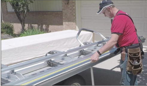
Create a 3/4" tab on one side of the over flashing
