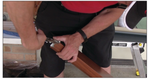
Create tabs for an adjustment of 2 pieces
