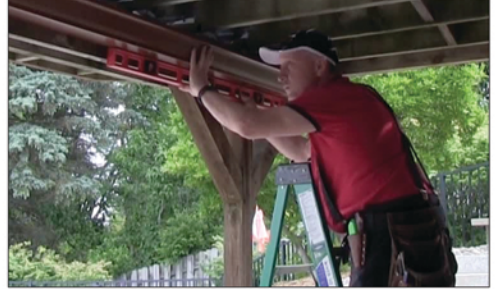
Set the pitch from the center to the low end
