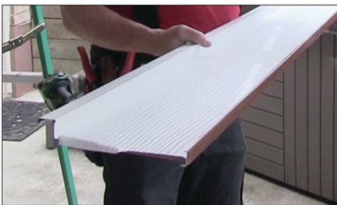
Create a “Twisted Tongue” on one Panel
