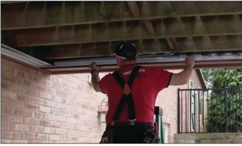
Slide the panel into the Gutter, G-Channel, and Side Cap
