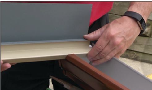
Check that the Side Cap fits snugly into the gutter
