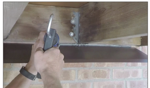
Seal the top of the Over Flashing
