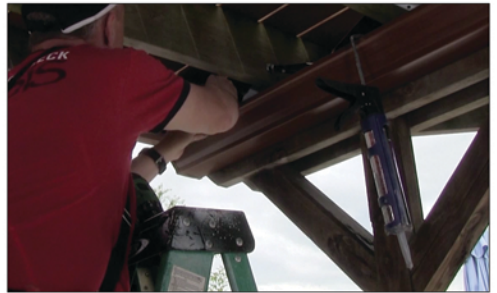
Put on the end cap and seal it
